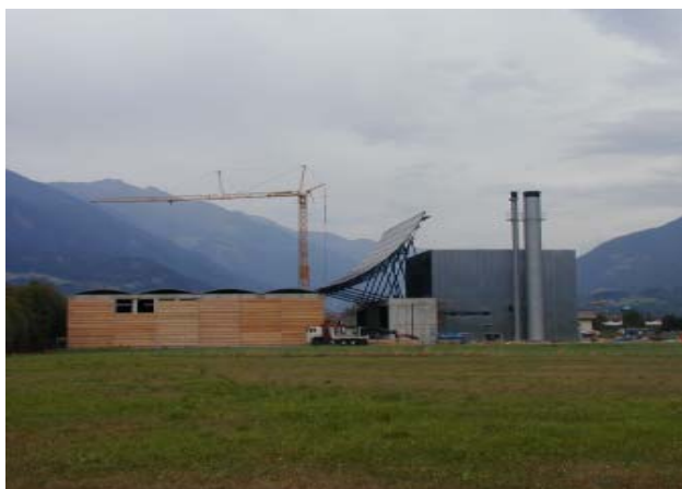
Figure 2.1: The wood-fired heat station in Lienz
